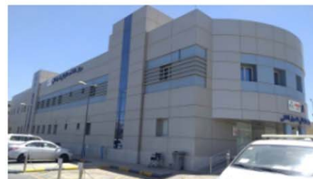
DIAVERUM DIALYSIS CENTER KHAMIS MUSHAIT_EXTENSION GENERAL CONTRACTING Mar 2018
