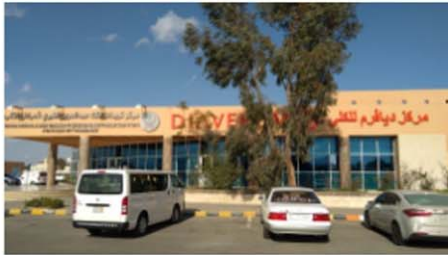
DIAPERUM CLINIC ABHA GENERAL CONTRACTING Dec 2017
