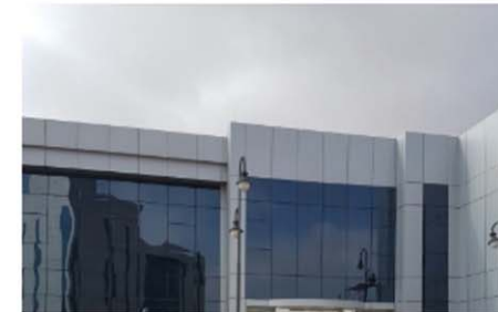
DIAPERUM DIALYSIS CENTER SAKKAKA GENERAL CONTRACTING Mar 2017
