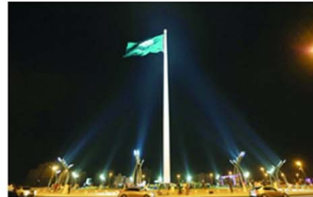
THE TALLEST FLAGPOLE IN THE WORLD - FLAG POLE SQUARE JEDDAH ELECTRO - MECHANICAL WORKS Sep 2014
