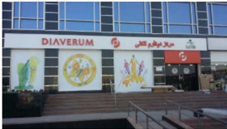
DIAPERUM CLINIC AL DAMMAM 9019 GENERAL CONTRACTING Dec 2016
